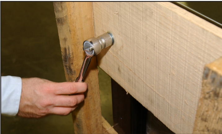
Removing skid from bottom of cabinet.
