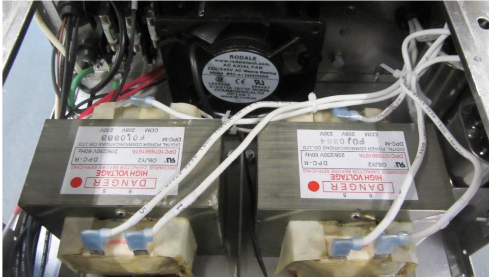
HIGH VOLTAGE TRANSFORMERS – COOLING FAN
